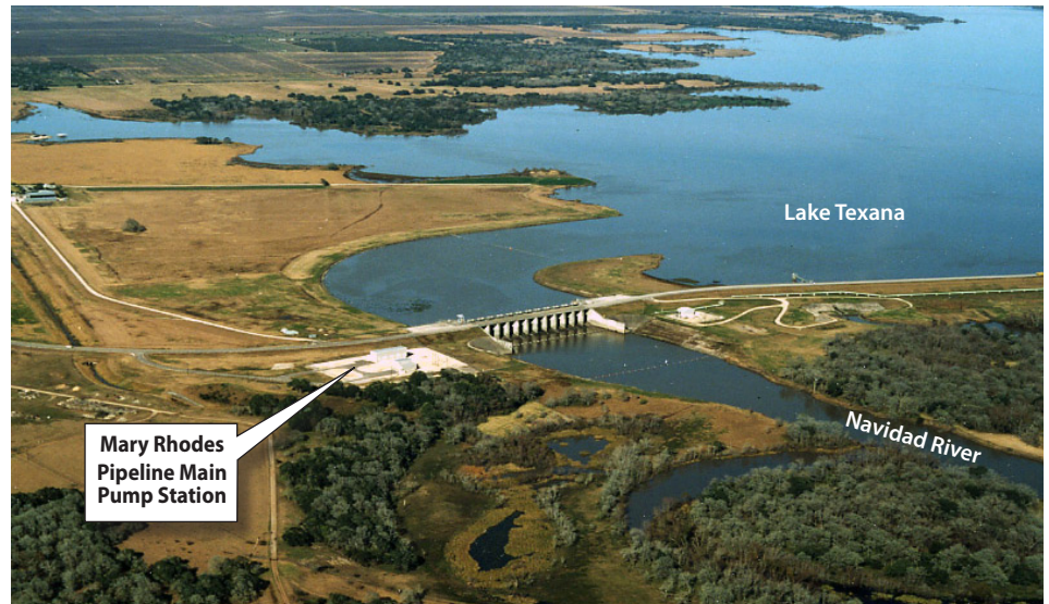
Palmetto Bend Dam creates the 11,000-acre Lake Texana in Jackson County. Lake water is delivered to Coastal Bend customers through the 101-mile long, 64-inch diameter Mary Rhodes Pipeline.
